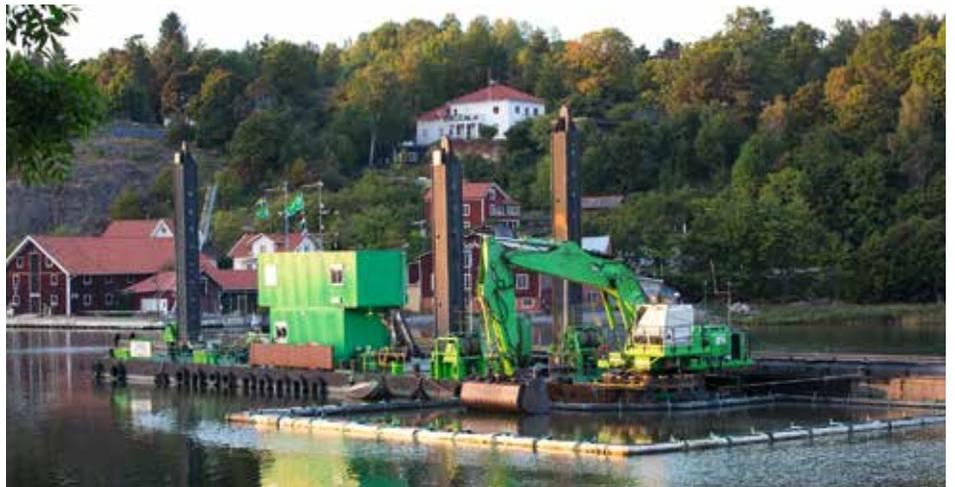
Figure 5. Because of the presence of contaminated sediments, environmental dredgers are tasked with having even greater accuracy than other types of dredging.
